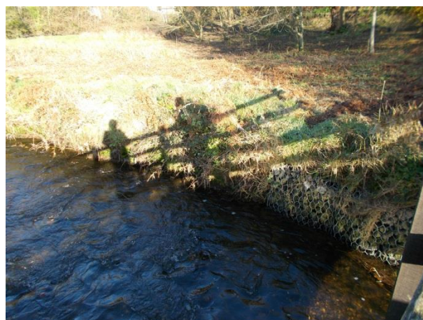
Figure 5.22: Gabion baskets along the right bank under a footbridge crossing the Afon Wygyr
