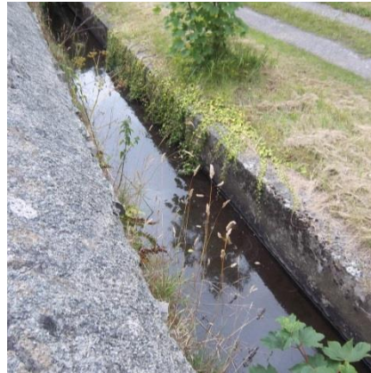
Figure 5.25: Bank and bed reinforcement on the Nant Cemaes
